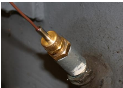
Transformer oil pocket with temperature probe installed.
