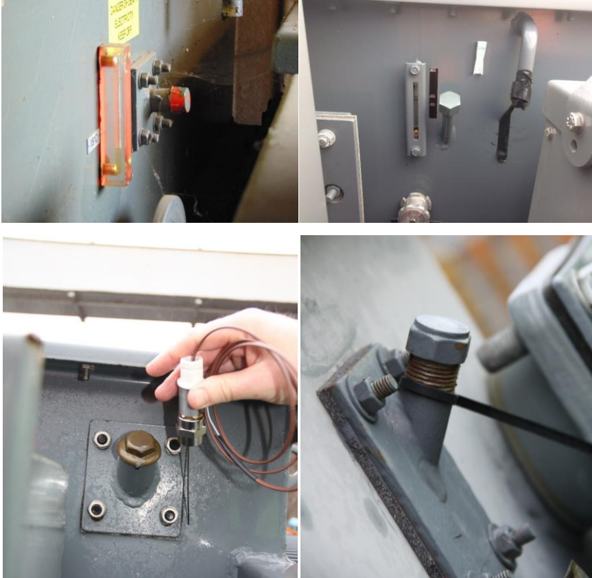
Transformer oil pocket with temperature probe installed.
