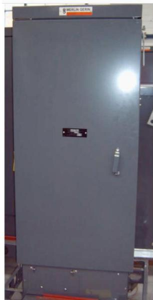
**Figure 1 - Merlin Gerin transformer mounted LV cabinet**
