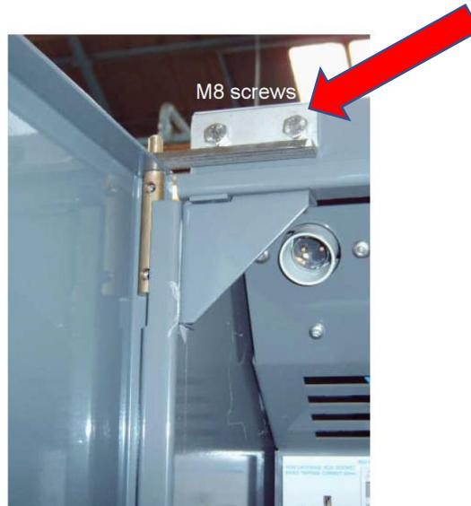
**Figure 5 - LV Cabinet door securing bolts**
